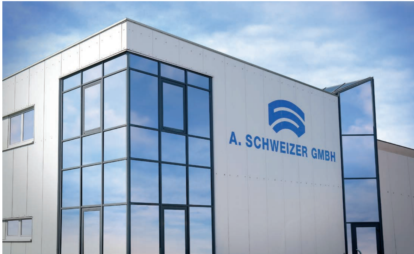
SCHWEIZER headquarters in Forchheim / Germany with a production area of 5500 m².
